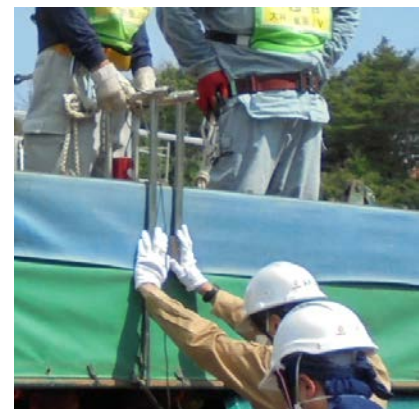
Fig.1 Measurement of the truck sidewall thickness
